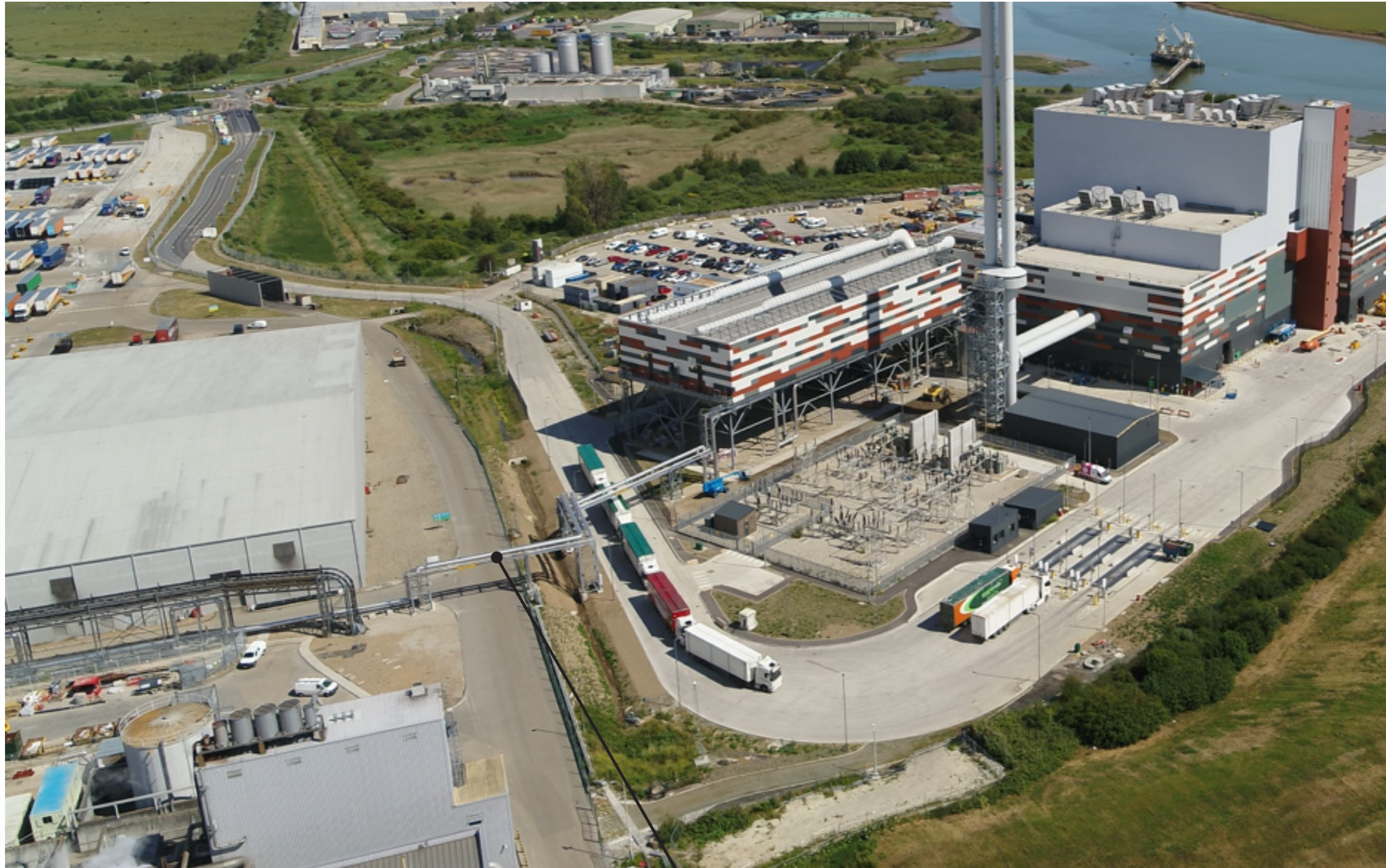
Steam connection pipebridge from K3 to the Kemsley Paper Mill
